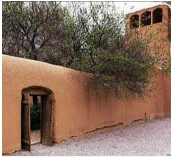
Figure 14- the landscape of architectural building in urban space
