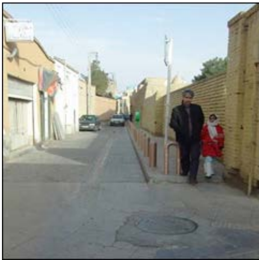
Figure 6: Separating the sidewalk from the roadway, a variety of flooring (Jolfa)
