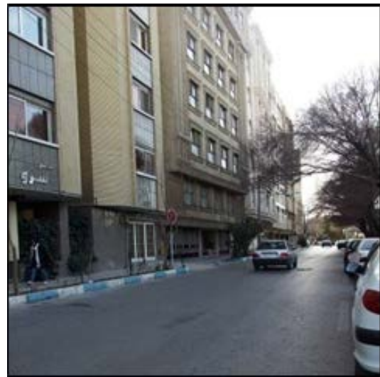
Figure 7: The newly constructed Sector (Jolfa)
